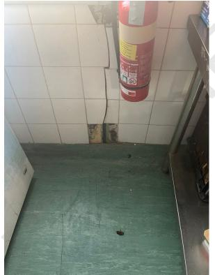
The floor beneath this freezer was significantly affected by the fire of 2020 and this freezer has obviously been placed over the affected area.
