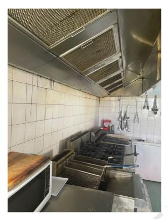
The wall and exhaust are in need of a proper and thorough cleaning.
