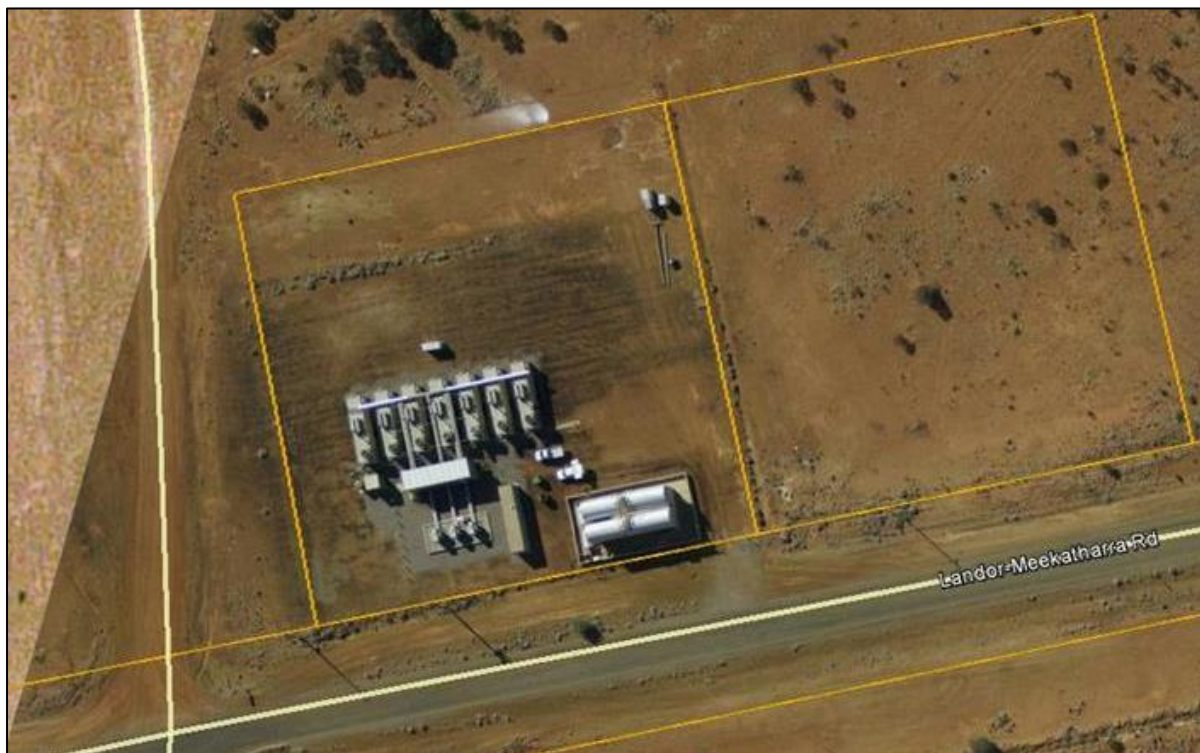
FIGURE 42 - MEEKATHARRA POWER INFRASTRUCTURE
