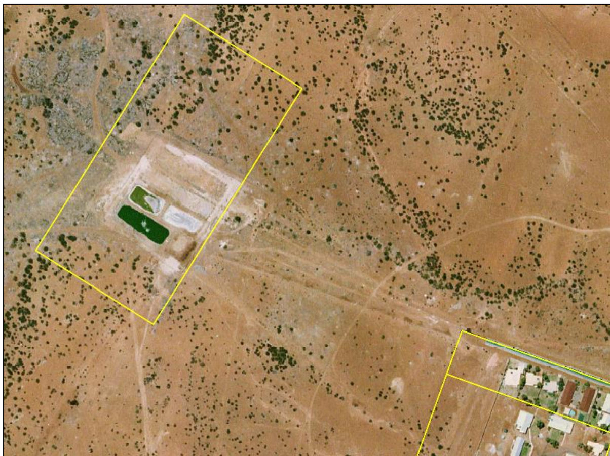
FIGURE 41 - MEEKATHARRA WASTEWATER SITE
