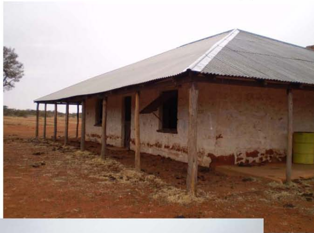
Old Mt Gould Police Station
