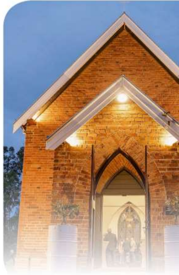
ABOVE: St John's Church, Pinjarra. Image by Josh Cowling Photography.
