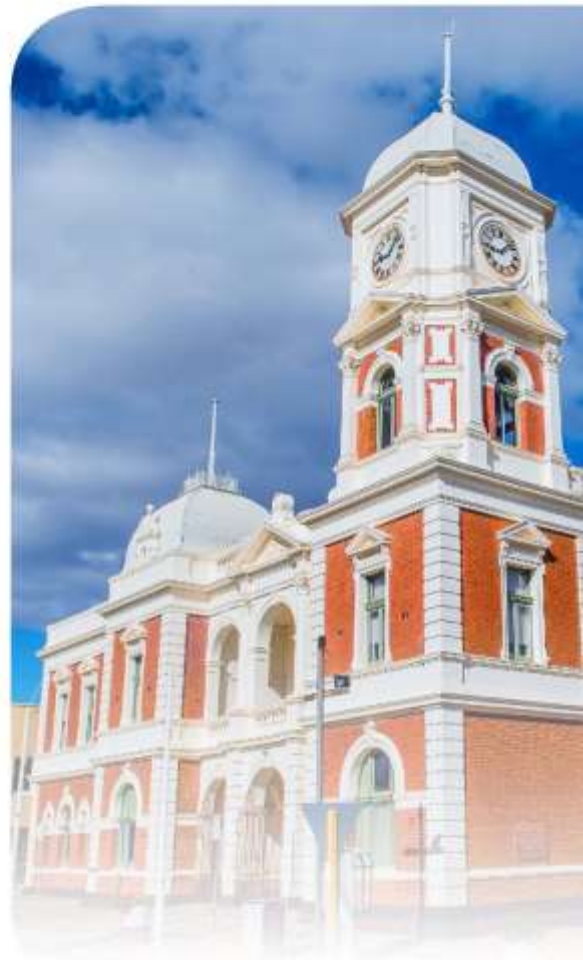
ABOVE: Boulder Town Hall. Image supplied by the City of Kalgoorlie-Boulder.
